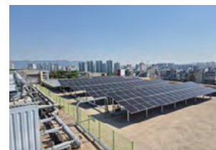
[LOTTE Shopping] Solar Panel Installation
