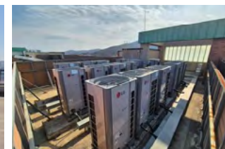
[LOTTE Department Store] High-efficiency Air Conditioner Replacement
